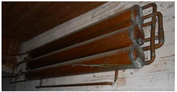
Coil of pipe for heating water
